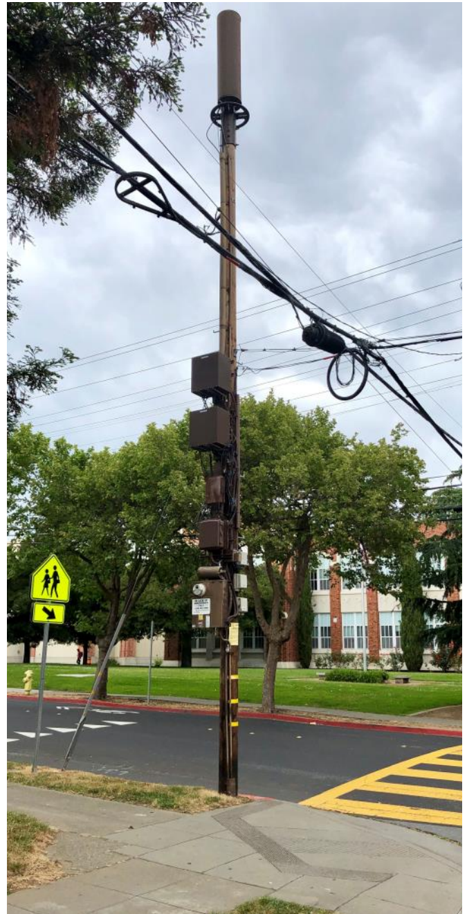
"Small Cell" equipment boxes and antenna added to existing pole in front of San Mateo High School
